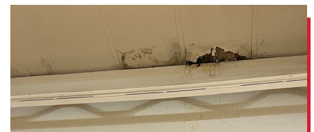
Deteriorating Gymnasium Ceiling
